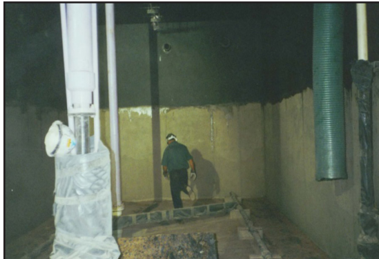
Concrete protected with ARC 791 and ARC 988
